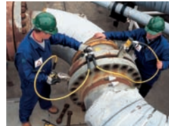
Two ENEFSH14 spreaders used simultaneously with Enerpac handpump & hoses.
