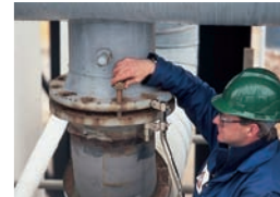
Flange alignment with ENEATM1
