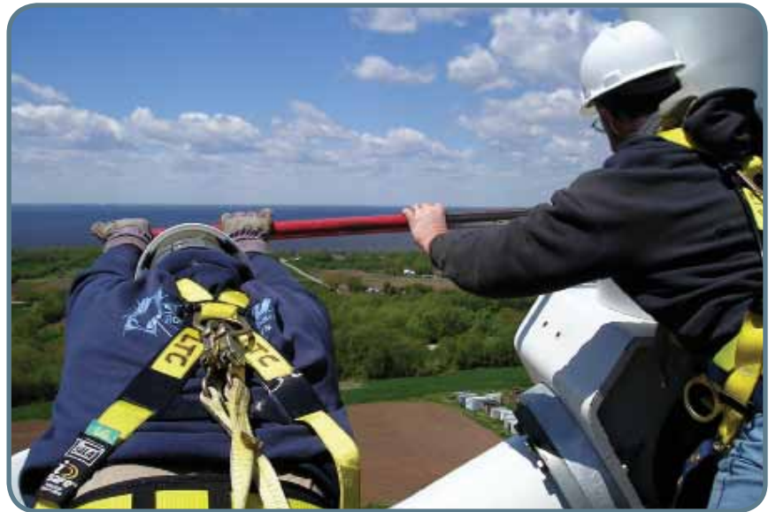
Former students of Doug Lindsey, Terry Hendrickson (left) and Joe Stalker, put their backs into their work tightening bolts on turbine blade.
